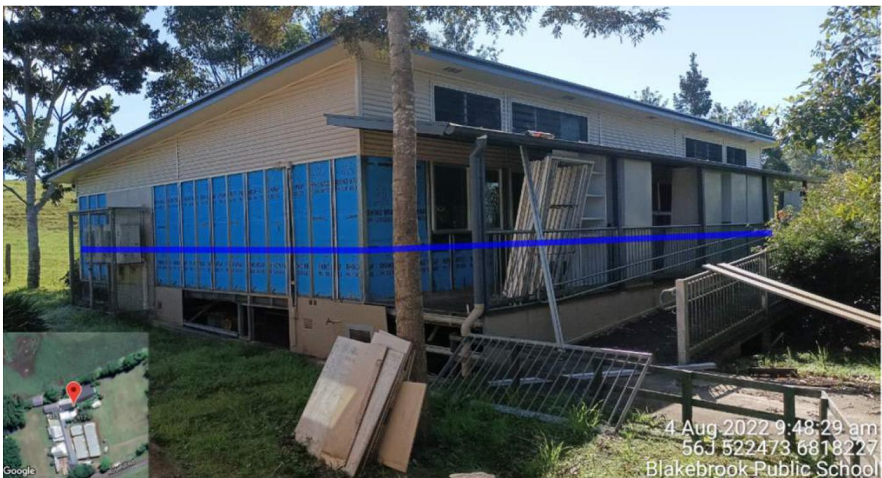
Figure 19: Building A learning spaces with Feb 2022 flood height indicated by blue line (Source: Acor Consultants)
