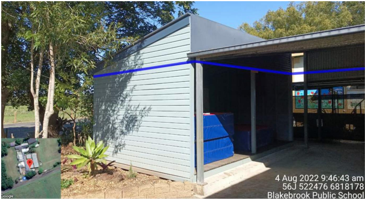
Figure 18: Storage building with Feb 2022 flood height indicated by blue line (Source: Acor Consultants)
